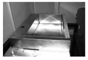
2. Place the blower unit in the well making sure to slide it flush against the wall of the well.
