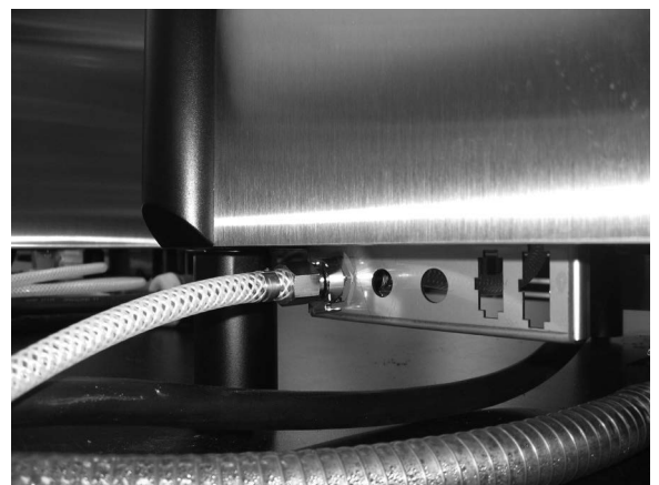
INSTALL WATER SUPPLY LINE
