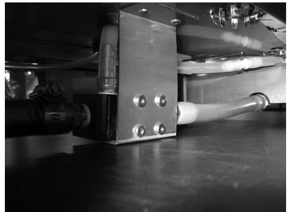
INSTALL DRAIN HOSES TO MANIFOLD
