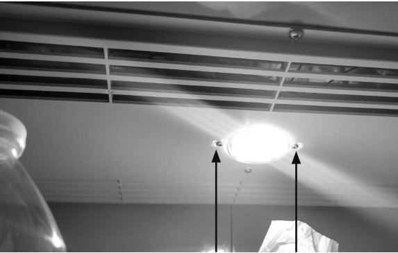
Two (2) Screws Secure the Light in the Unit
