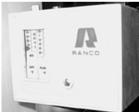
Thermostat located behind the On/Off switch panel.
