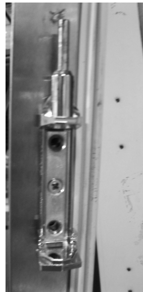
Photo 2. Rotate hinge 180°
