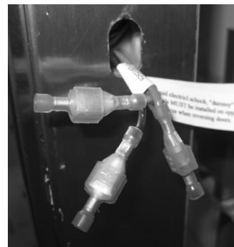
Photo 3. Remove the caps and reinstall them on the opposite side switch wires
