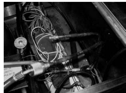
Pressurize the low side to 250 PSIG [17.2 Bars] using nitrogen, check for leaks and pressure level after 10 minutes & again after 24 hours.
