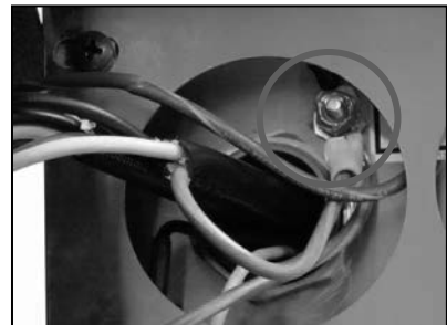
Remove top ground connection from main front ground post.
