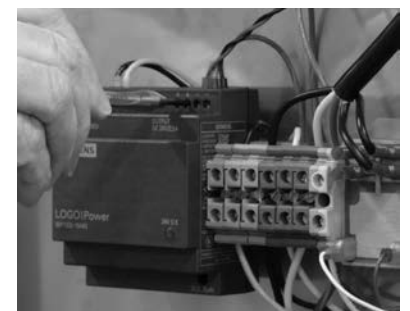
Use small screwdriver to release high & low voltage wires from Power Supply.
