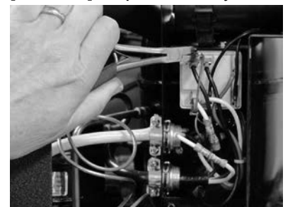
[Photo 4] Replace Relay
