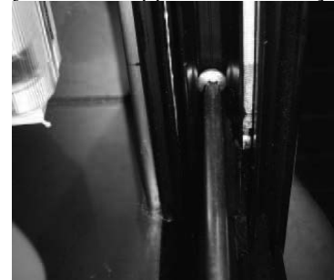
[Photo 5– Upper Track View]
