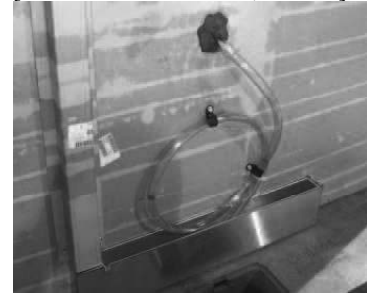
The condensate collection heater is located under and behind center of case bottom.
