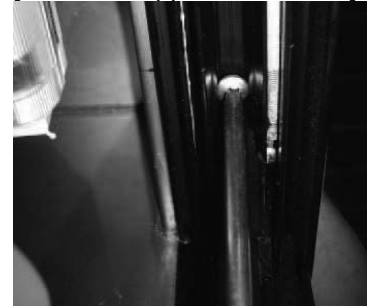
[Photo 5– Upper Track View]
