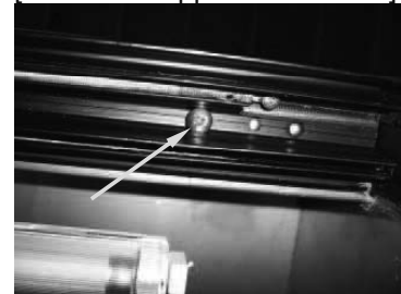
[Photo 4 – Upper Track View]
