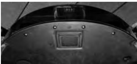
Example of top repair
