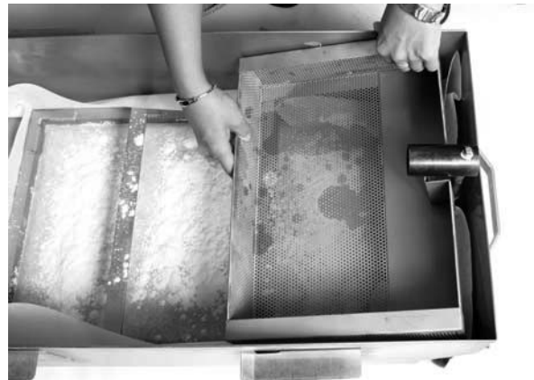
Crumb screen properly placed.
