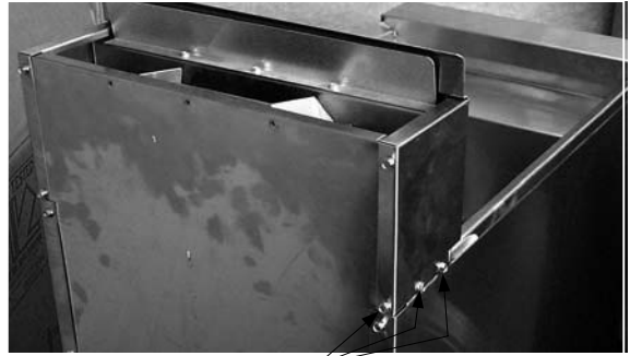
Three screws, on each side of the fluecap, must be removed.
