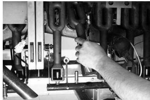
Remove burners to gain access to temperature probe.
