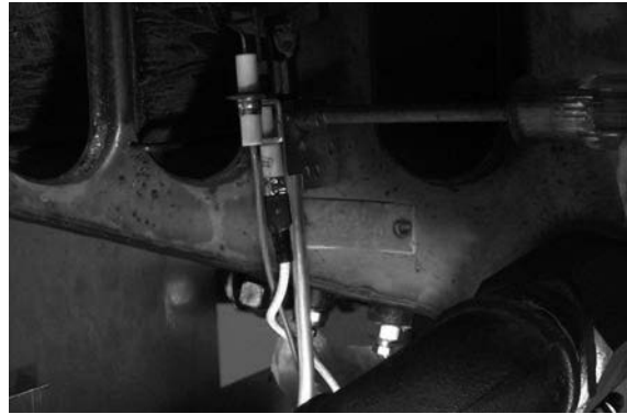
Removing electronic/standing pilot assembly.
