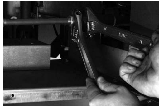
Holding backup while unscrewing flare nut on oil-return line.
