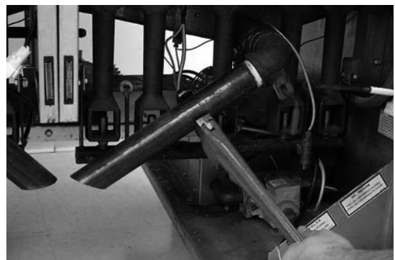
Removing 1.5" drain extension. (Step 19.A)
