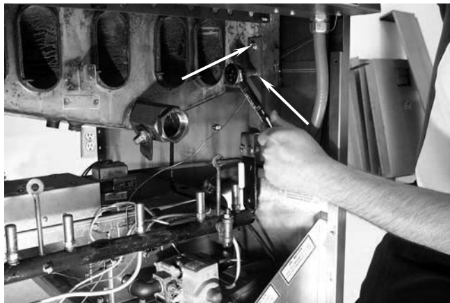
Removing bolts (arrows) from burner manifold support brackets (both sides). Leave the burner manifold in place after removing bolts.
