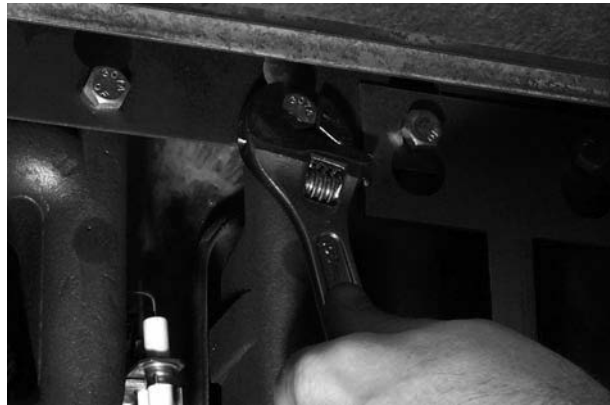
Loosening burner bolts prior to burner removal.
