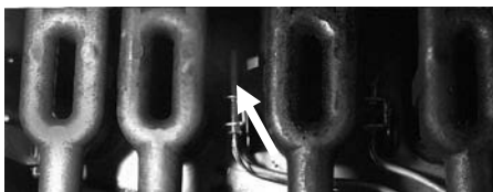
Position of standing pilot (arrow) on unit with that feature.
