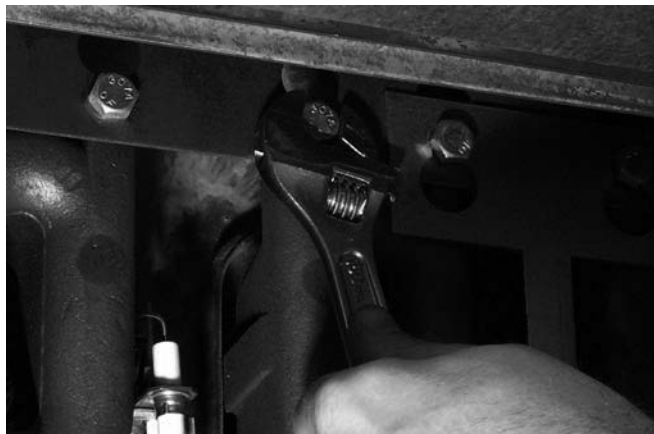
Loosening burner bolts prior to burner removal.
