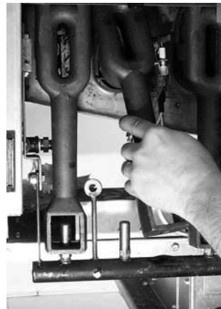
Removing burners from rethermalizer.
