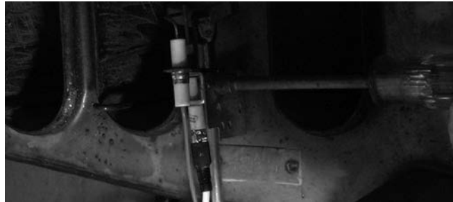
Removing electronic/standing pilot assembly.
