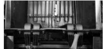
Fig: 10-13 Hardware on fixed elements in sub fryer.
