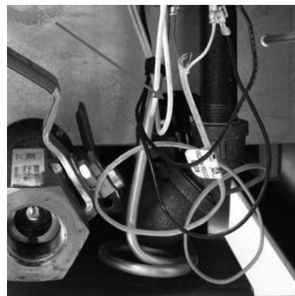
Insert match or taper through this hole to light pilot.
