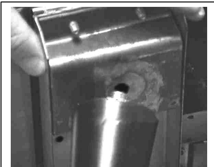
INSTALLING LEG INTO LEG SUPPORT ASSEMBLY
