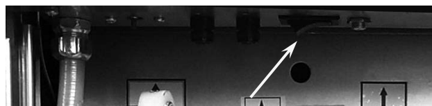
After the hose/wand end is properly positioned in the frypot, activate the filter pump with the auxiliary switch inside the cabinet (arrow).
