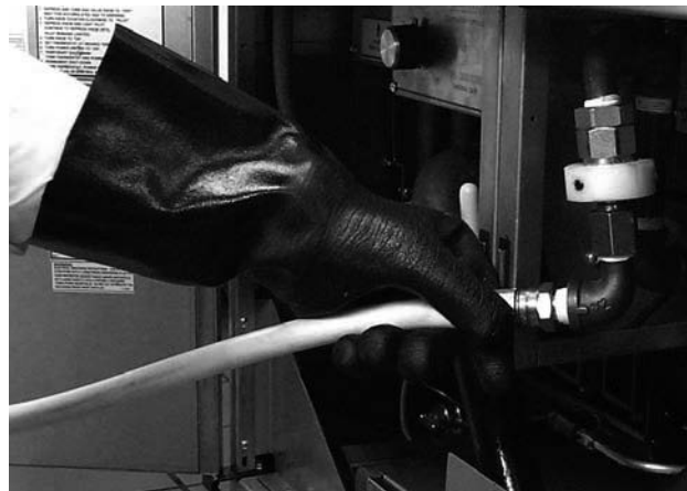
Hose/wand disconnect properly connected to disconnect valve in fryer cabinet.
