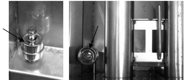
Figure 1: The float switches (above and right) should be cleaned periodically to eliminate starch buildup, which can impede the motion of the floats. Take care, however, to ensure the shafts are not dislocated or the movement of the float hindered.
