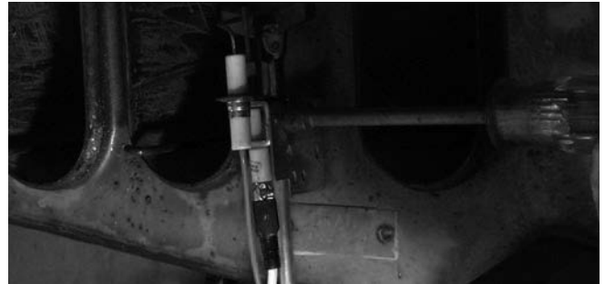
Removing electronic/standing pilot assembly.
