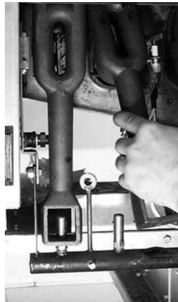
Removing burners from rethermalizer.
