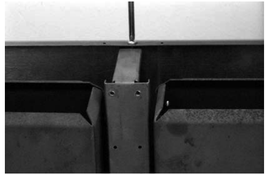
Removing brace holding back panel to flue cap.
