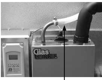
Install and insulate glycol line from heat exchanger to bath
