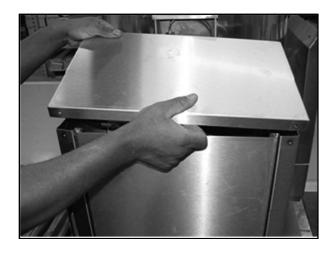
1.3 Assemble the riser to the new pedestal cover as shown below, installing the gasket directly under the cover and then the backing plate.
