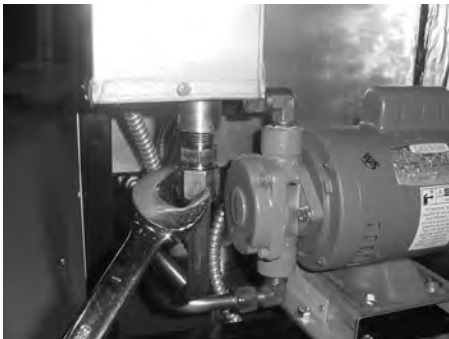
Condensation Box Fitting Step 1
