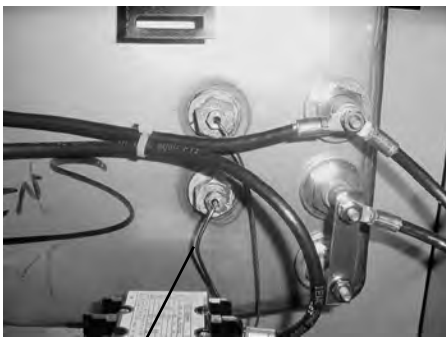
High Limit Capillary Tube
