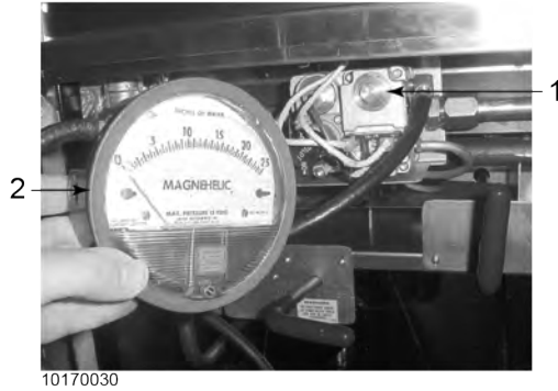
Figure 2-15 Adjusting Regulator
