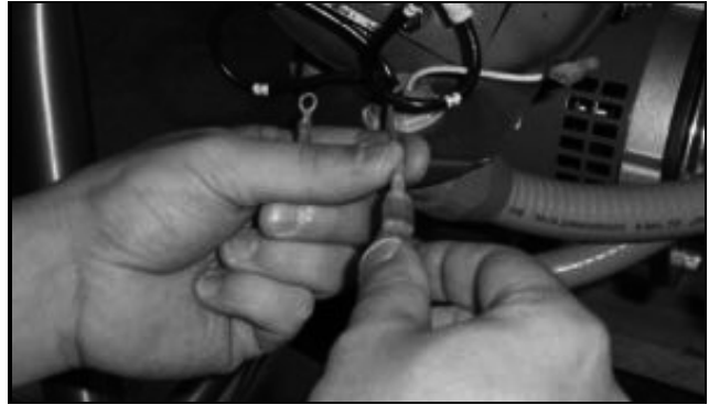
Attaching the jumper wires.
