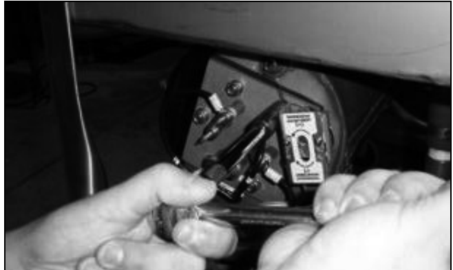
Removing the thermostat bracket/heater nuts.
