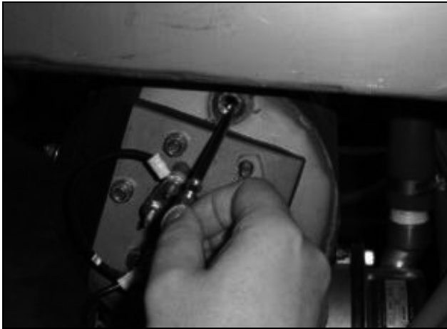
Pulling the thermostat probe and fitting from the well.
