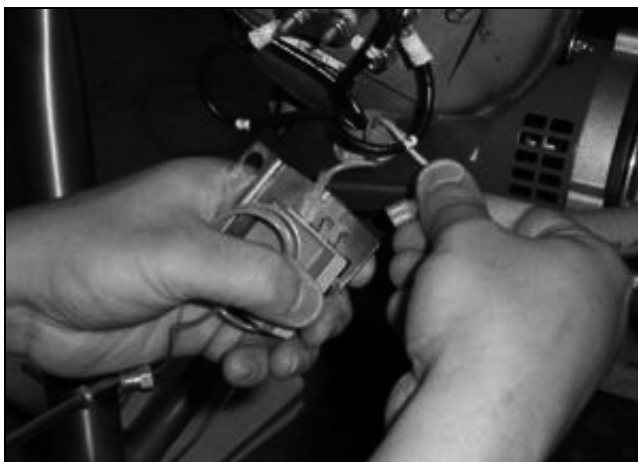
Removing the wires from the thermostat.
