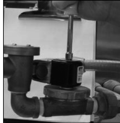
Removing the top screw
