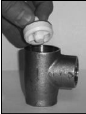
Removing the plunger
