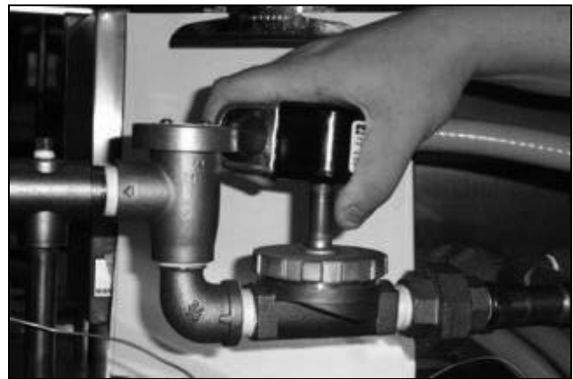
Removing the coil
