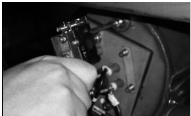
Putting the new thermostat in the well.
