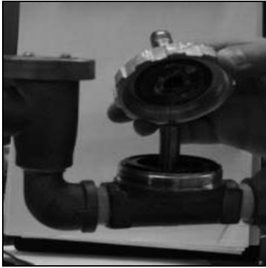
Removing the valve bonnet
