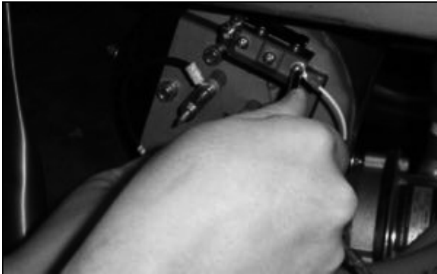
Securing jumpers to the thermostat.
