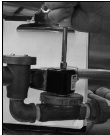
Removing the top screw
