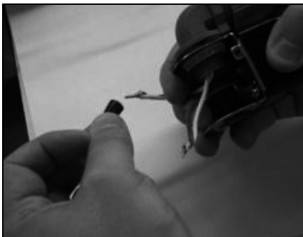
Removing the wire nuts
