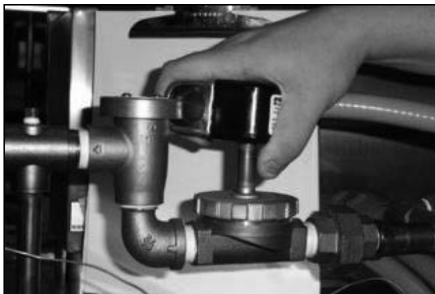
Removing the coil
