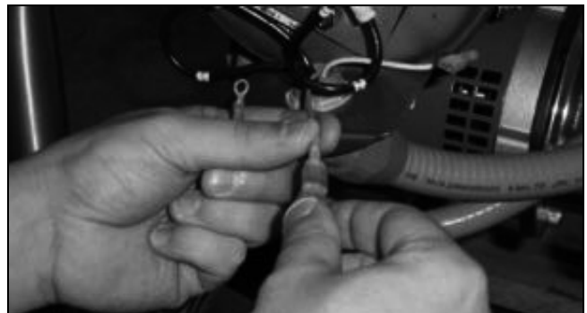
Attaching the jumper wires.
