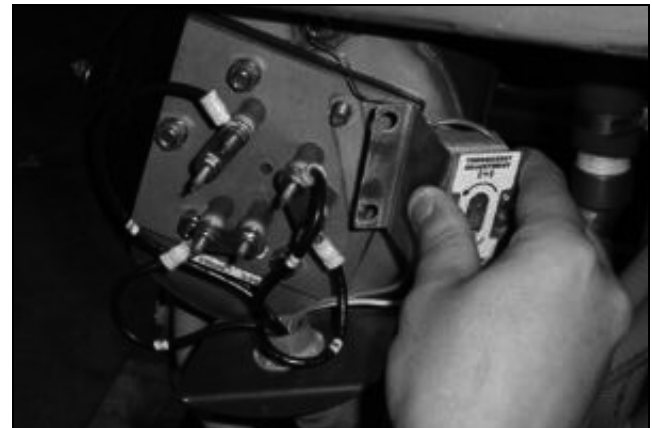
Removing the thermostat bracket.
