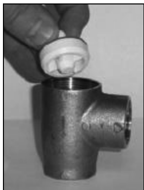
Removing the plunger
