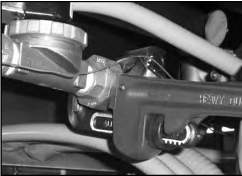
Loosening the union on the incoming plumbing
