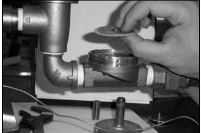
Removing the diaphragm
