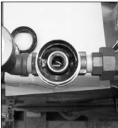
View inside the solenoid valve body
