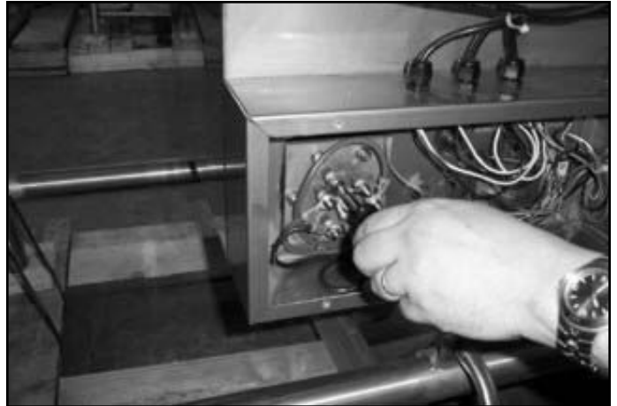
Removing the power lines.
