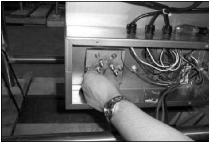
Removing silicone from thermostat well
