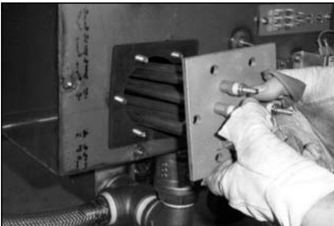
Removing the heater
