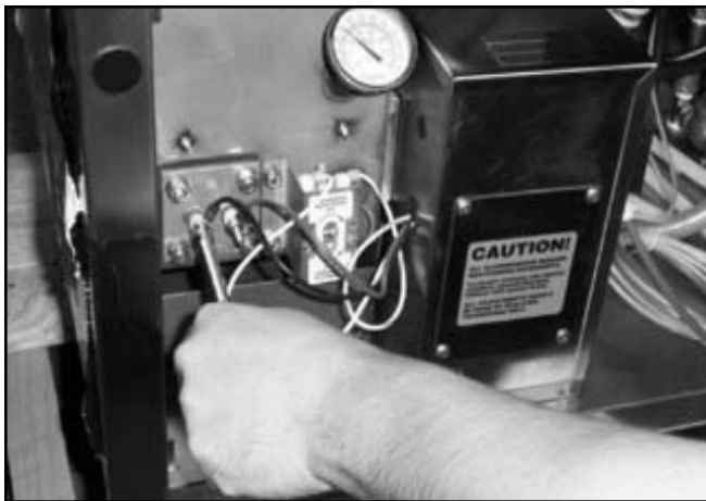
Removing the heater nuts.
