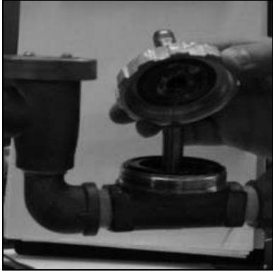
Removing the valve bonnet
