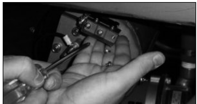
Removing the thermostat screws.
