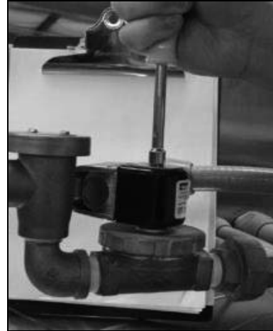
Removing the top screw
