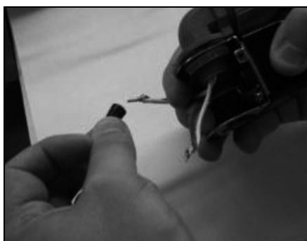
Removing the wire nuts
