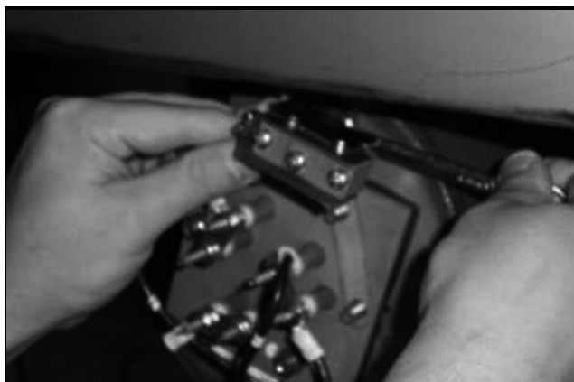
Tightening the brass fitting (Tempstar).
