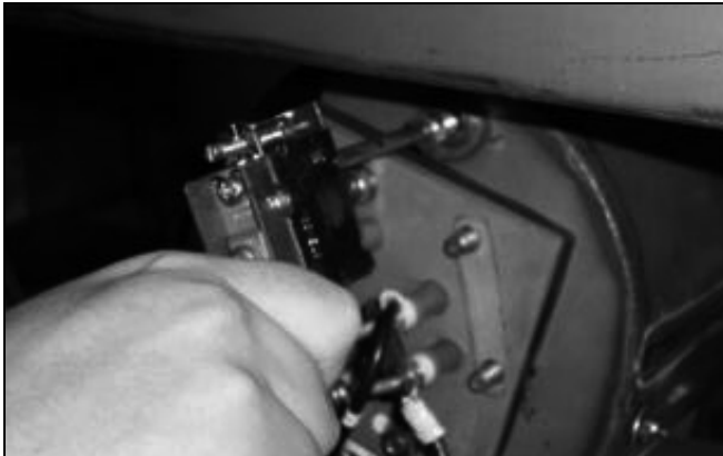
Putting the new thermostat in the well (Tempstar).
