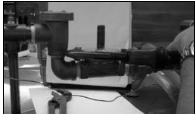
Loosening the valve bonnet
