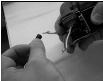
Removing the wire nuts
