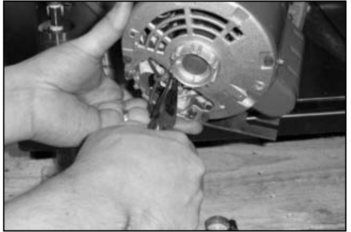
Removing the power wires.
