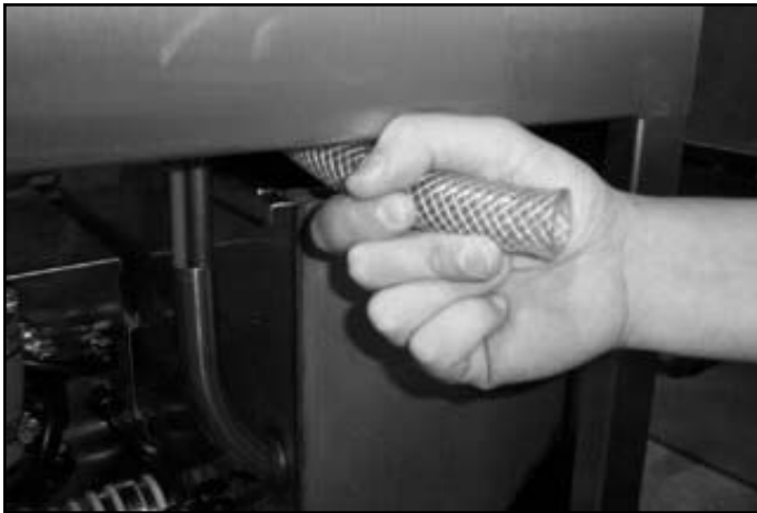
Pulling the discharge hose out.
