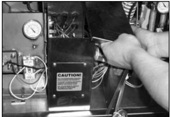
Removing the electrical box cover.
