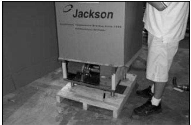
Lift the box off of the unit.
