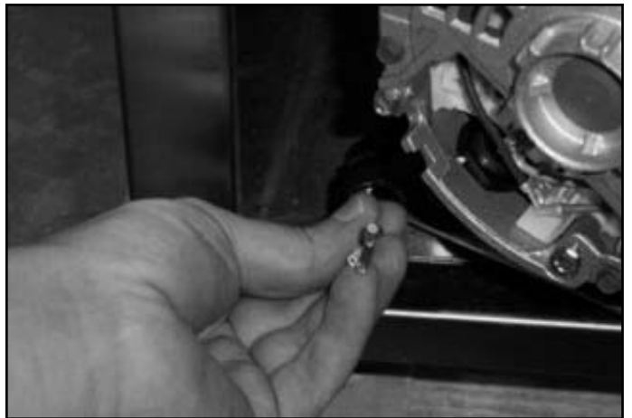
Removing the power wires.
