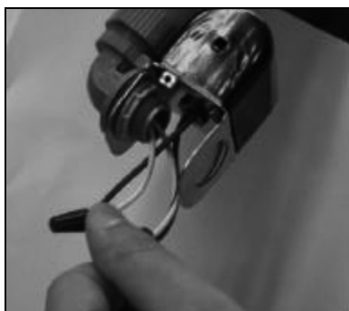
Straightening the wires
