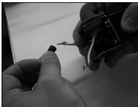
Removing the wire nuts
