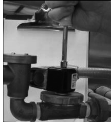
Removing the top screw
