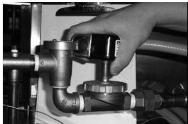
Removing the coil
