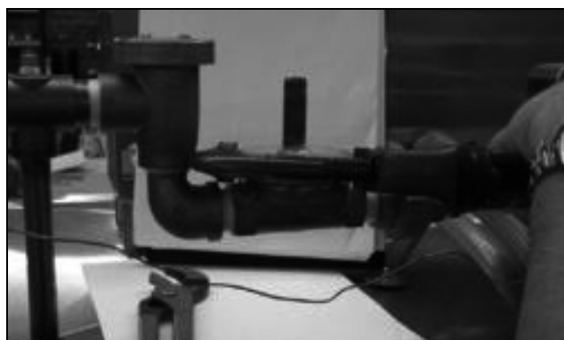
Loosening the valve bonnet
