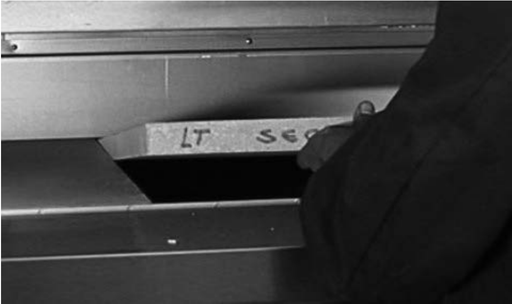
Bottom tile shown in position on "T" bar. FIGURE 1
