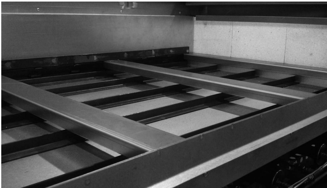
Bottom tile deck support channels running from front to back.
