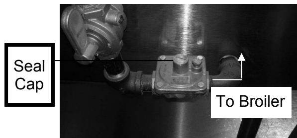
Figure 13. Gas Pressure Regulator
