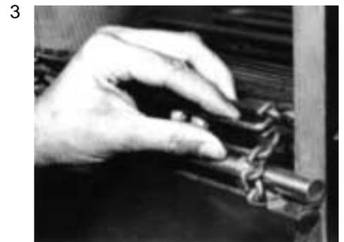
To reassemble, reverse the procedure. Be sure to reassemble the belt with the knuckle opening facing away from the direction of travel.
