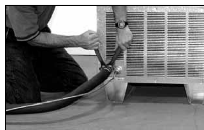
Connecting to the Condensing Unit Side
