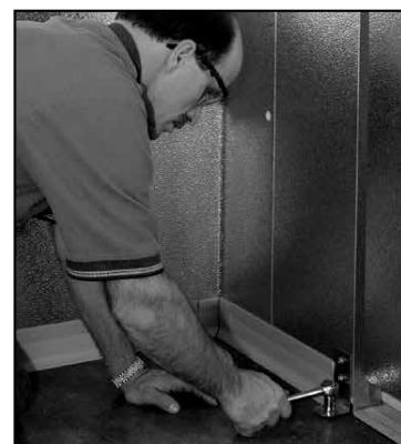
Attach slam brace with fastener provided
