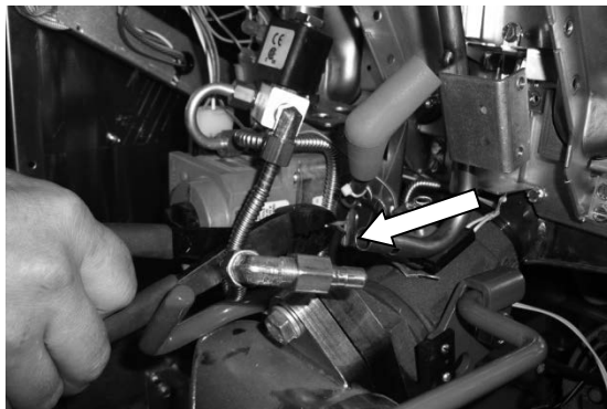
5. Change the SCB orifice tip.
