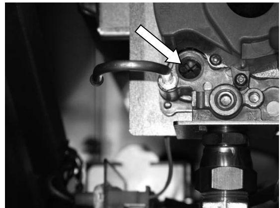
7. Adjust the burner manifold pressure. See section 26.2 “Taking a manifold gas pressure reading”.
