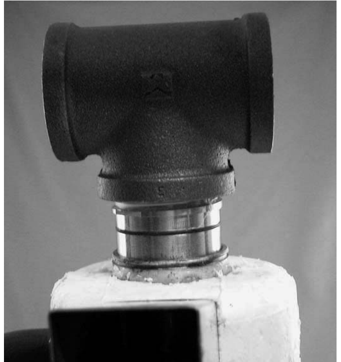
Tee Attached and Auger Lifted
