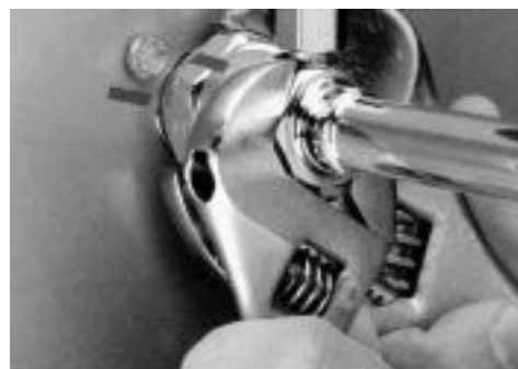
Rotate Swivel Nut 1/4 Turn More
