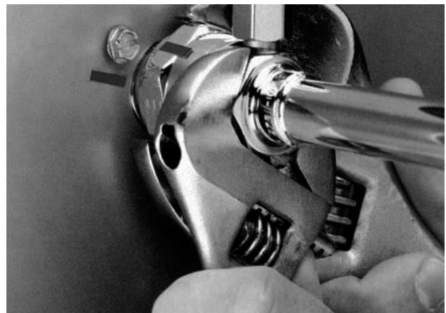
Rotate Swivel Nut ¼ Turn More
