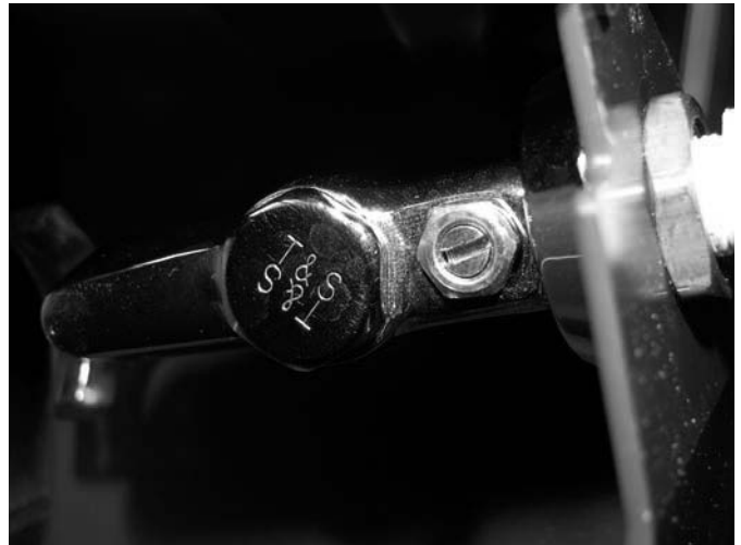
Water Flow Adjustment Screw
