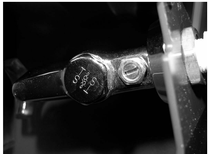
Water Flow Adjustment Screw
