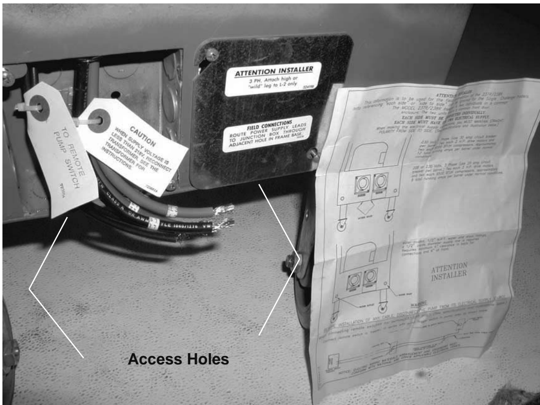
Figure 3 Electrical Connections
