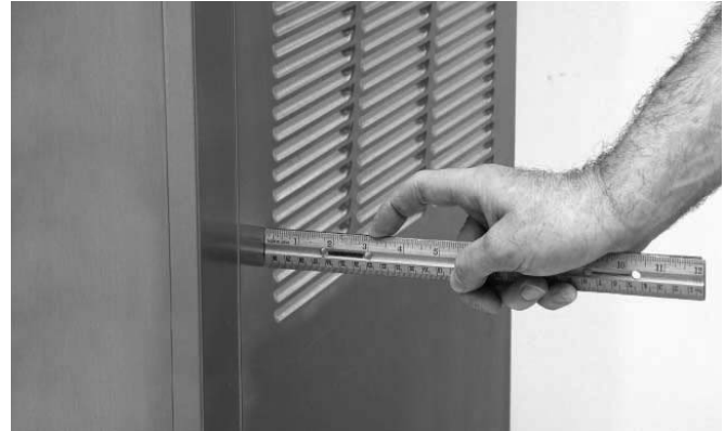
Figure 2-1 Space and Ventilation Requirements
