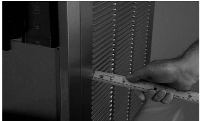
Figure 5. Space and Ventilation Requirements
