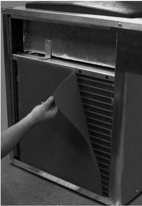
Figure 3-8 F112 Condenser Filter Removal
