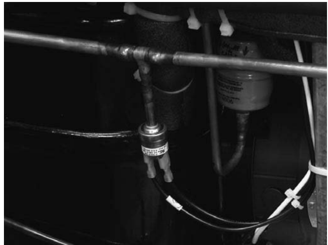
Figure 5-6 High Pressure Cutout
