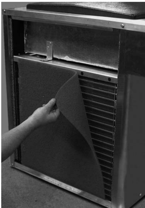
Figure 3-11 F112 Condenser Filter Removal
