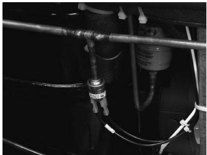
Figure 5-6 High Pressure Cutout
